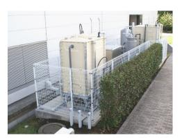
Groundwater membrane filtration system installed at the company's premise
